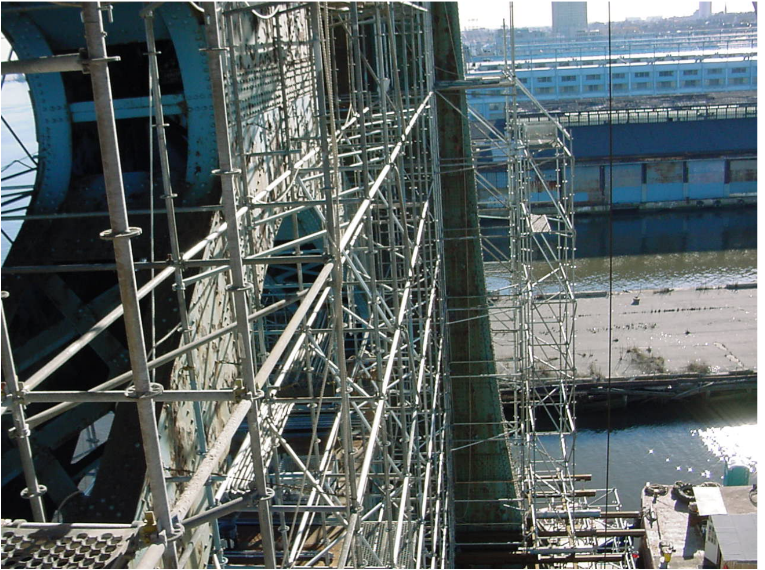
Scaffolding Installation Tower Base To Roadway
