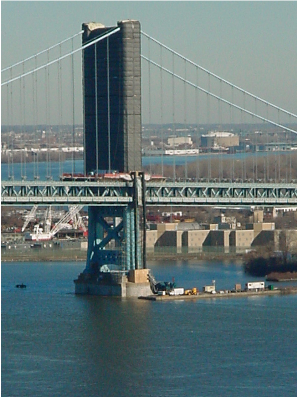
Scaffolding & Containment Around Camden Tower
