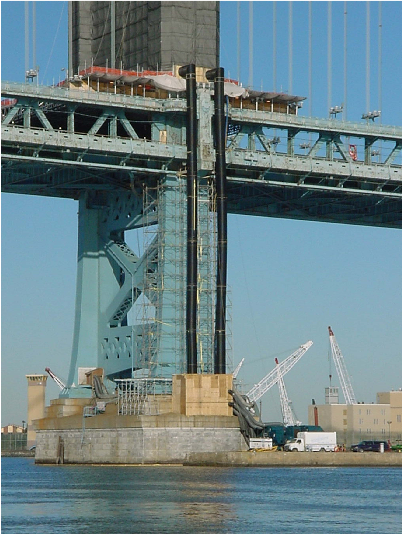
Scaffolding Installation Tower Base To Roadway
