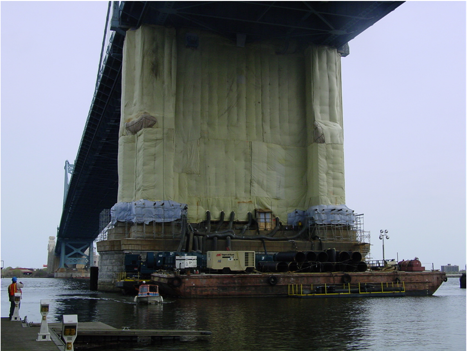
Containment Installation Around Scaffolding Tower Base To Roadway
