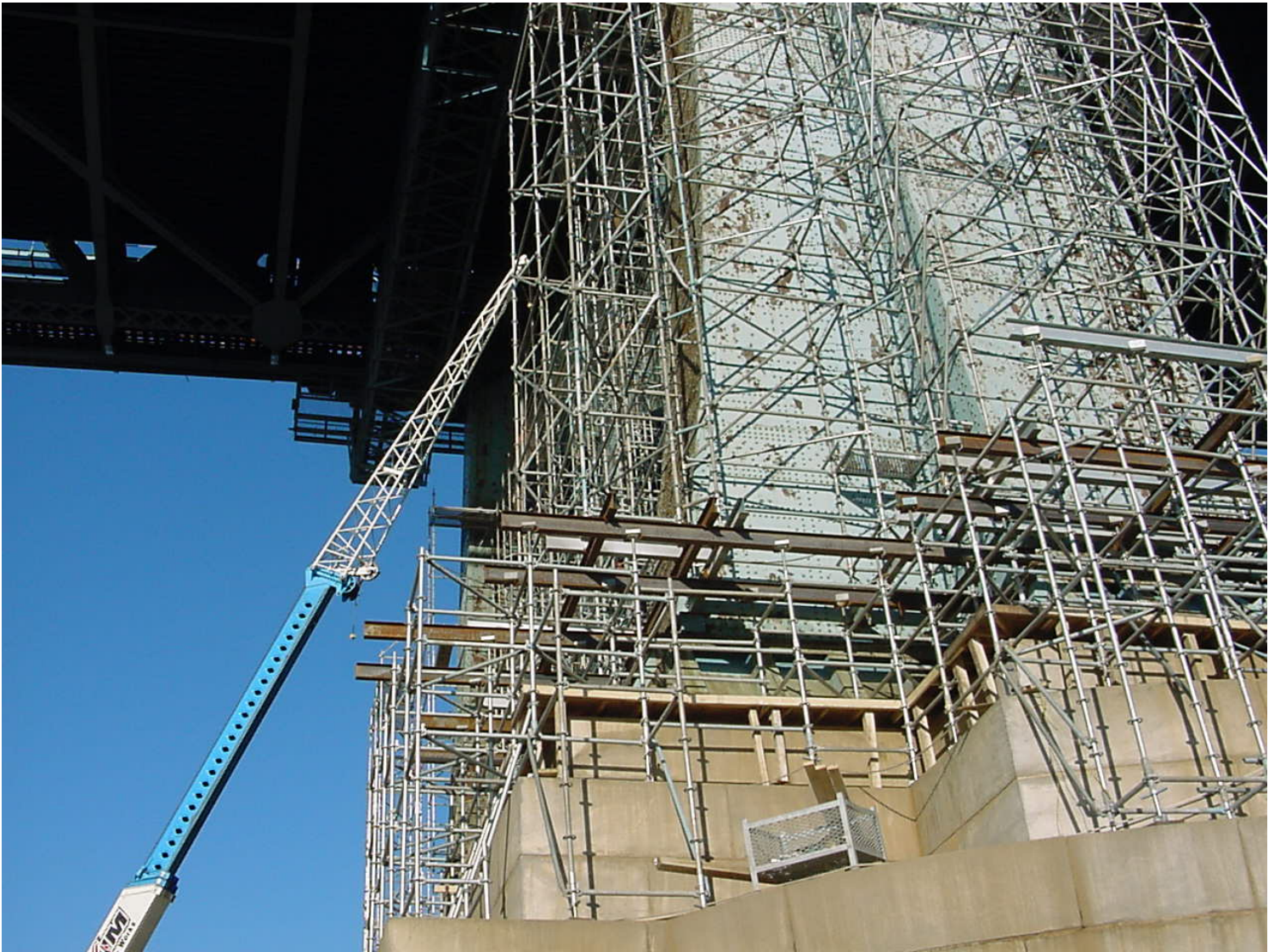
Scaffolding Installation Tower Base To Roadway
