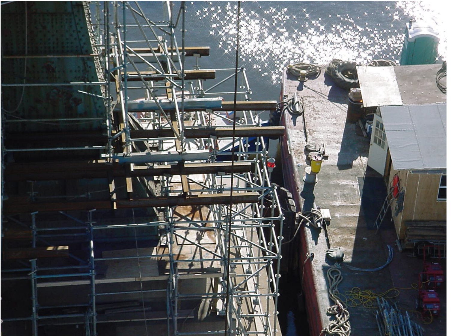
Scaffolding Installation Tower Base To Roadway
